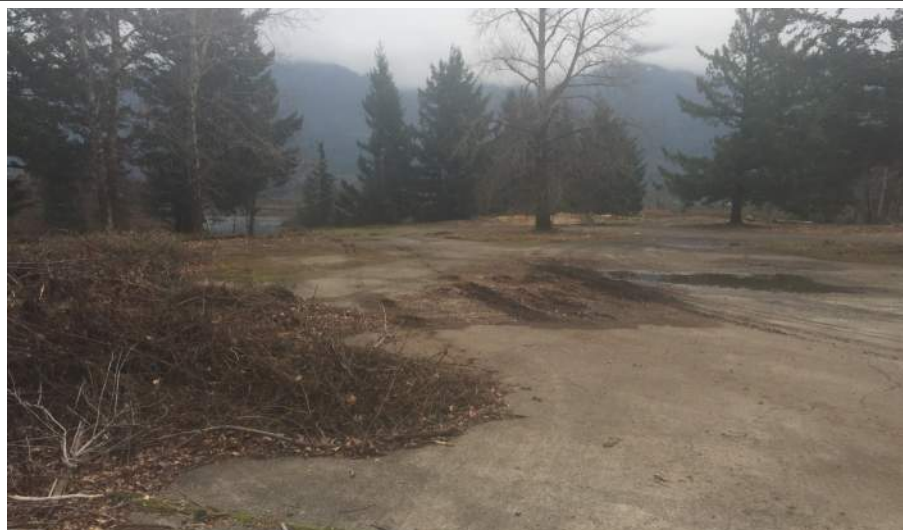
Photo 1. Existing concrete and gravel surfacing.
