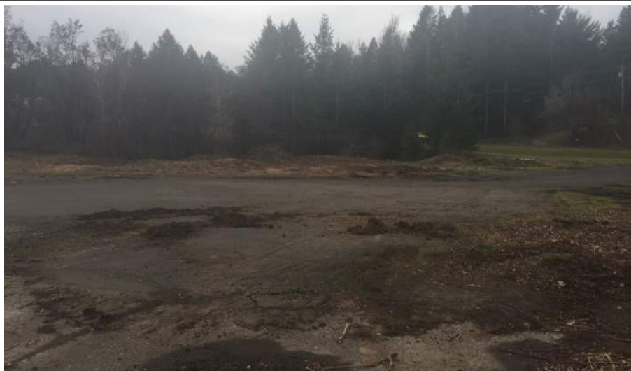
Photo 2. Existing concrete and gravel surfacing.
