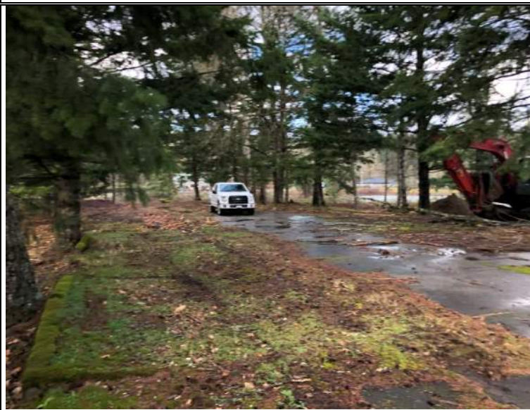
Excavation of test-pit TP-6, looking north
