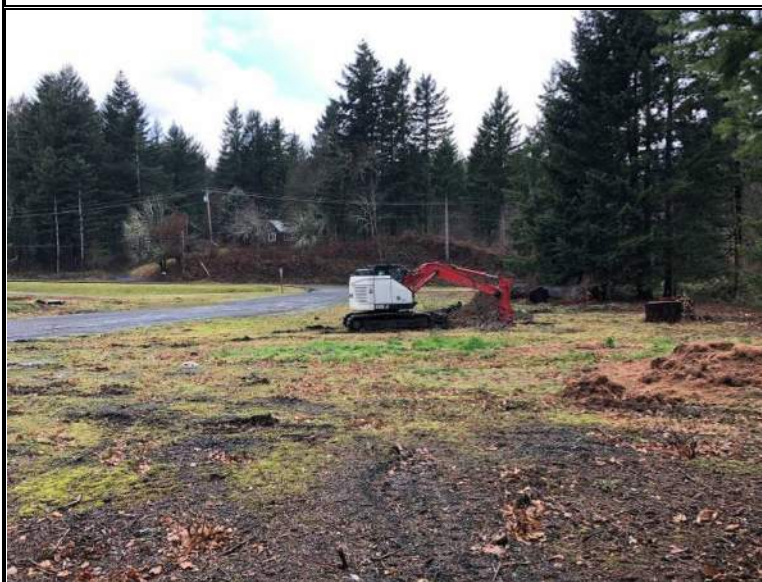
Excavation of test-pit TP-3, looking west
