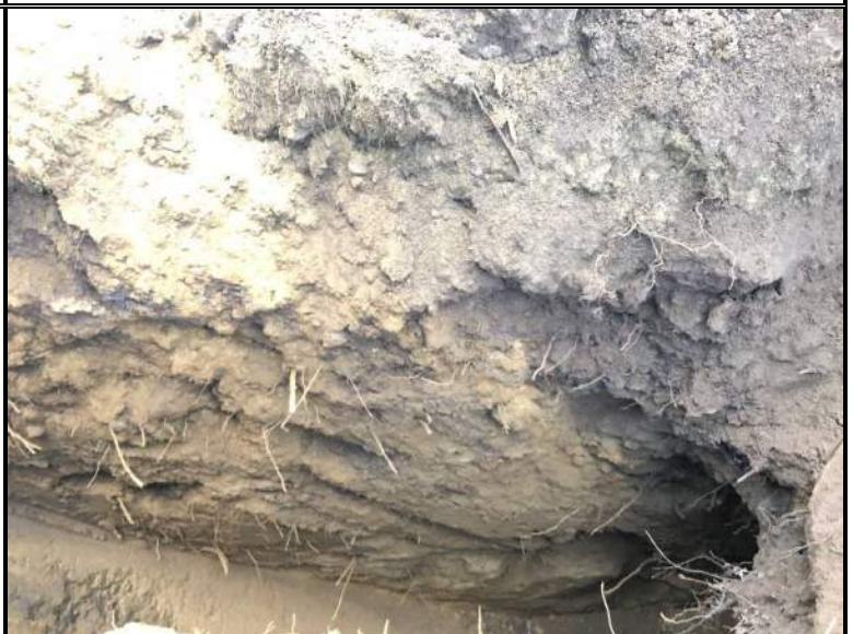
Exposed subsurface soil profile within test-pit TP-10
